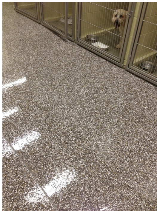
Kennel - Epoxy-Shell 1000 Full Chip Broadcast - Dark Earth
