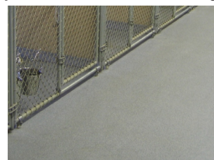
Kennel - Epoxy wall system Epoxy Quartz Floor - Slate
